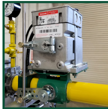
Honeywell Modutrol Actuator with Eclipse Butterfly Control Valve
