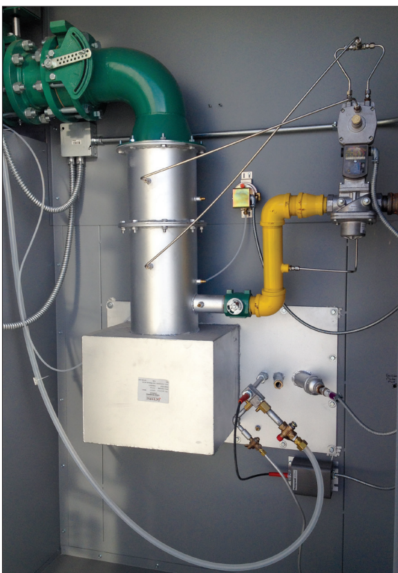
Linnox ULE burner installed inside the air handling unit.
