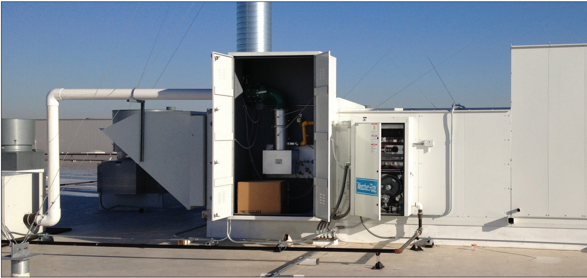
WEATHER-RITE™ make-up air handling system with Linnox ULE burner.
